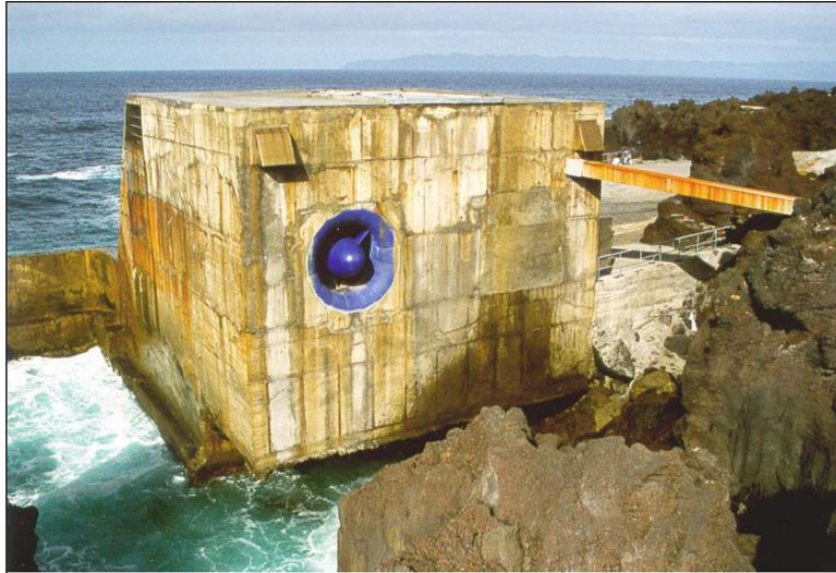
Figure 10: Pico plant WEC device
